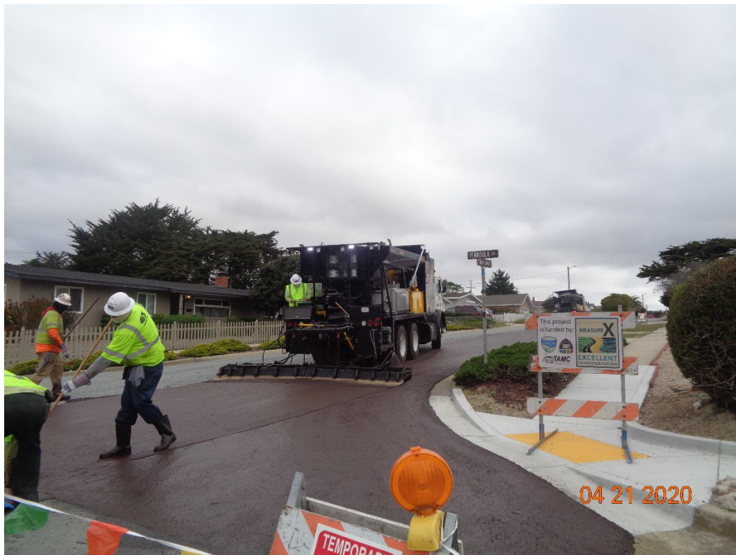
Figure 6 - Final Slurry Coating (Step 3)
