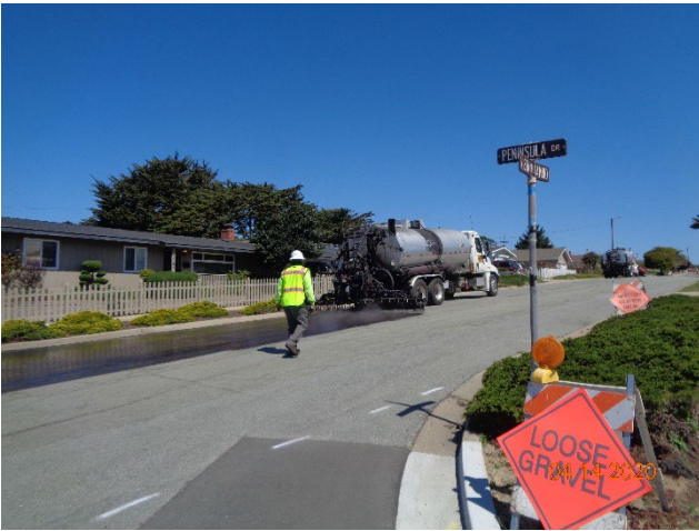
Figure 4 - Tack Coating (Step 1)
