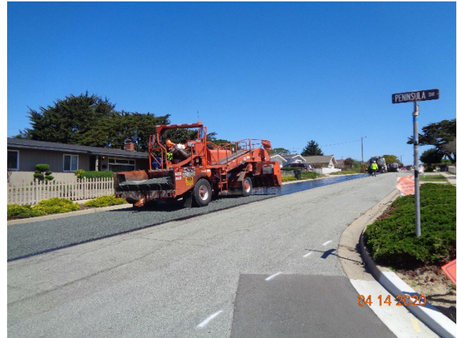
Figure 5 - Spreading Chip Aggregate (Step 2)
