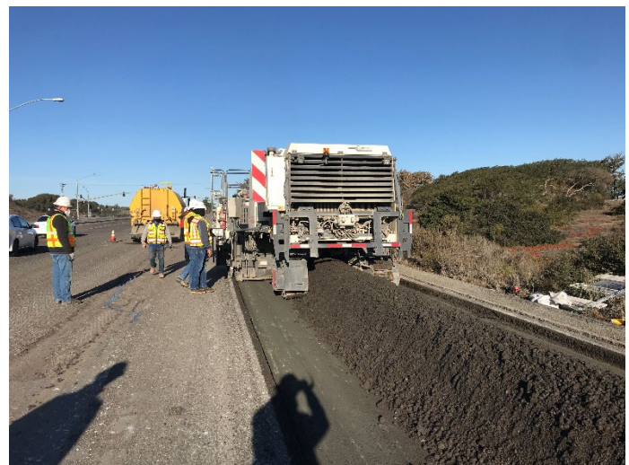
Recycled of pavement grindings
