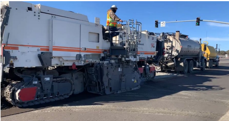
Front of CIR Train – Emulsion, Water & Grinder (11/9/2020)
