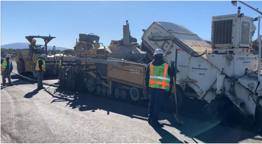
Rear of CIR Train – Paving Machine & Roller
